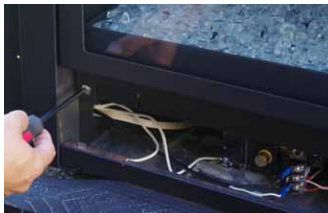
Figure 21. Remove lower left Door retaining screw.
